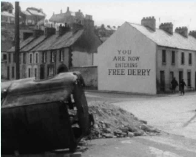
IRELAND – BEHIND THE WIRE (1974).
